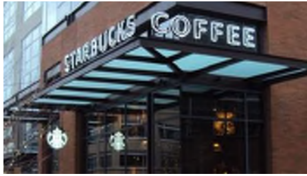
USTOM GLASS AND METAL CANOPY
